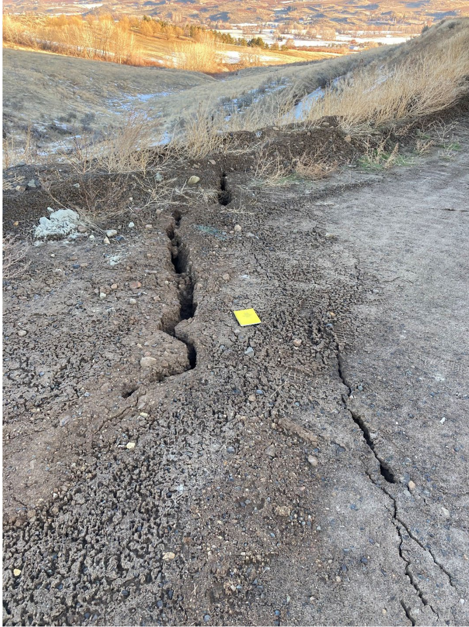
Figure 4: Cracks on perimeter landfill road.
