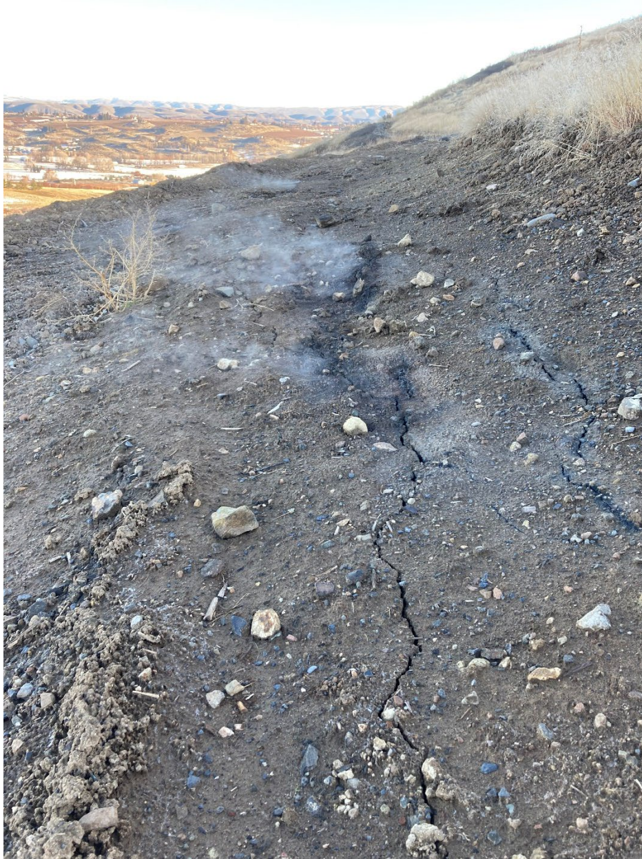
Figure 10: Facing north. Fine cracks in upper road above repaired slope with black residue around cracks and smoke/vapor emanating from cracks.
